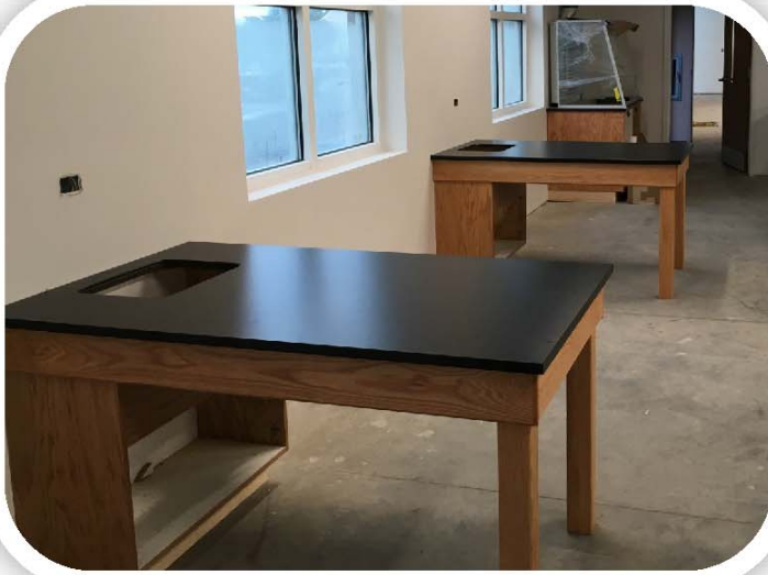
Lab benches installed
